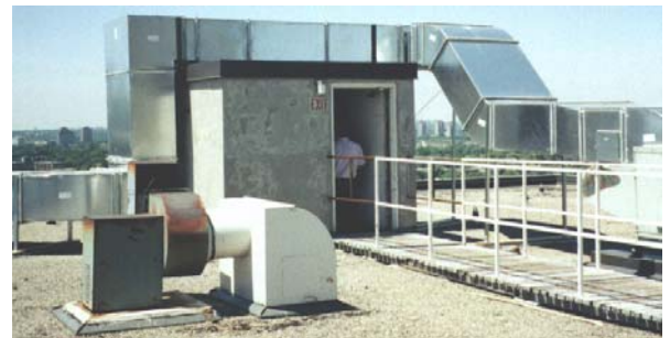
Duct connects to back of SolarWall panels (above). Duct passes over stairwell to connect to fan on north side of roof (below).
