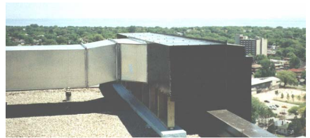
Duct connects to back of SolarWall panels (above). Duct passes over stairwell to connect to fan on north side of roof (below).
