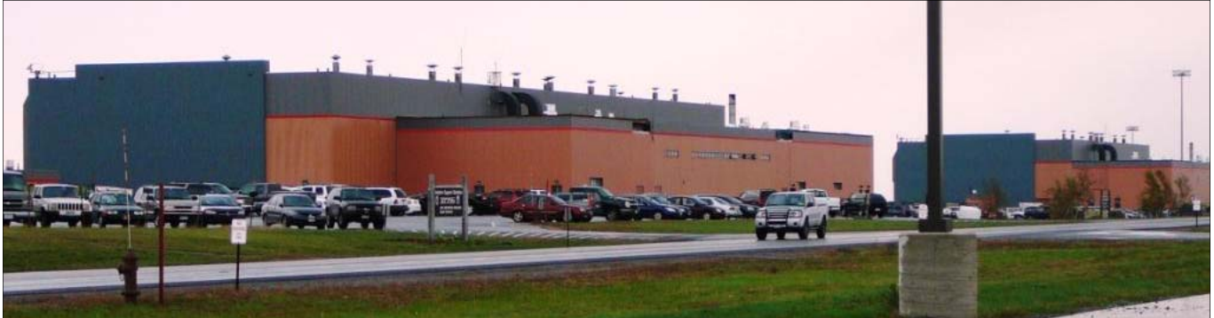
The world's largest collection of solar air heated buildings is located at Fort Drum, New York
