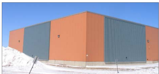
Blue-grey solar cladding installed on the south-east and southwest walls of Building 60.
