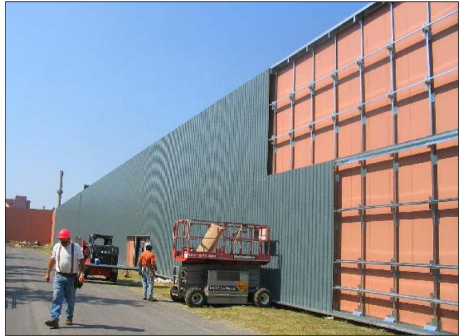
Above, the SolarWall panels being installed on the framing
