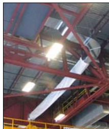
In buildings with heat stratification at the ceiling, the SolarWall system was connected to wall mounted fans and perforated distribution ducting to disperse the hot air at the ceiling around the building.
